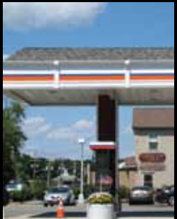
Gas Station Canopies
